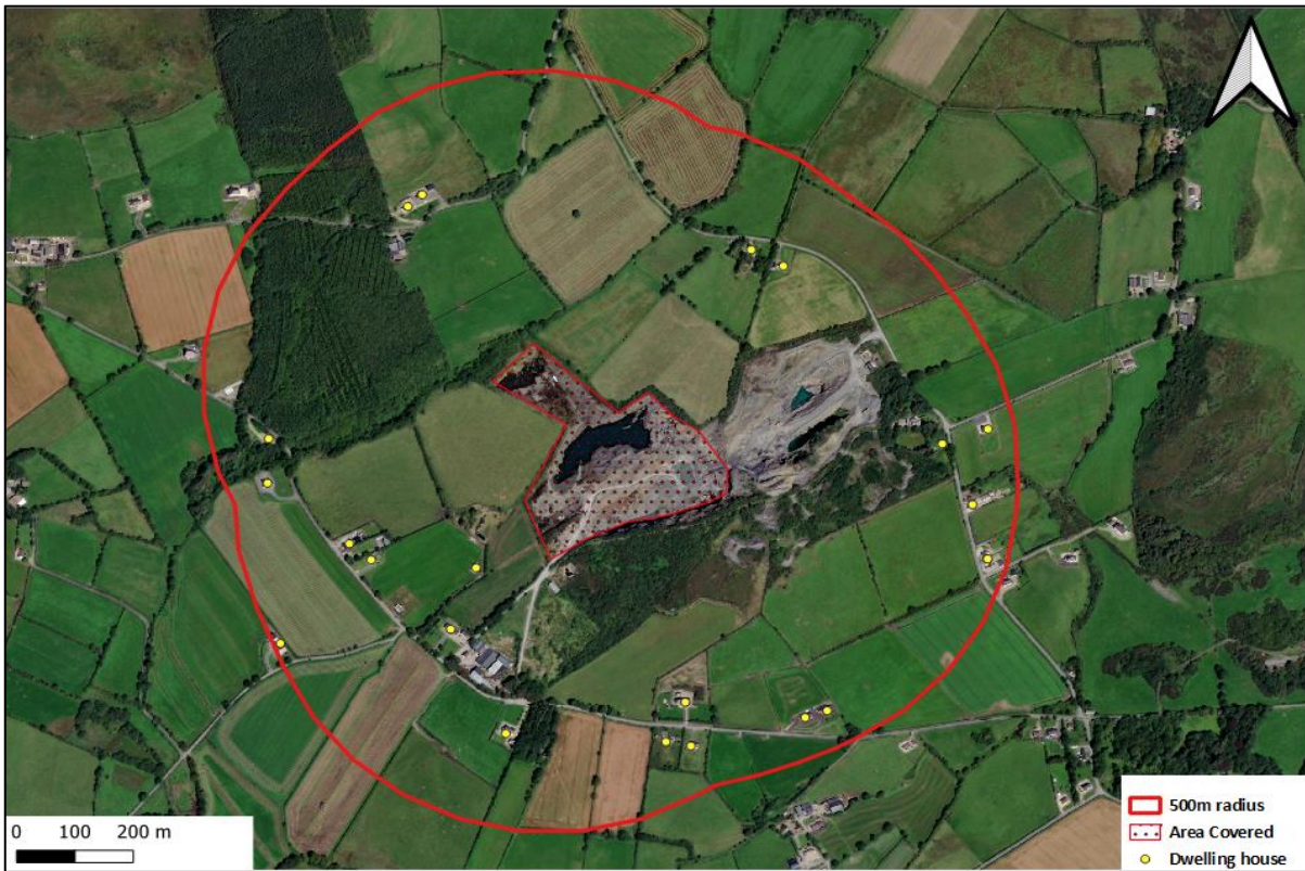
Image 5.2 Occupied Houses within 500m of perimeter of existing and proposed quarry
